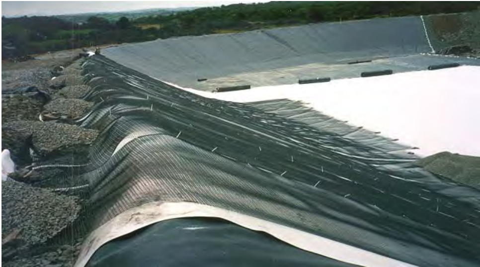
Plate 5.6 An Engineered Landfill Site Under Construction
